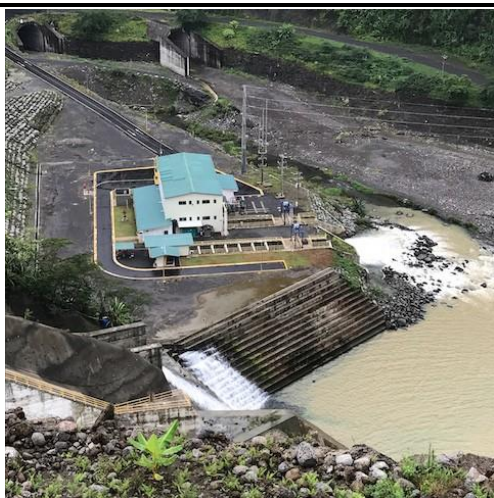
Photo 183: I-20 Ecological powerhouse (view from above)
