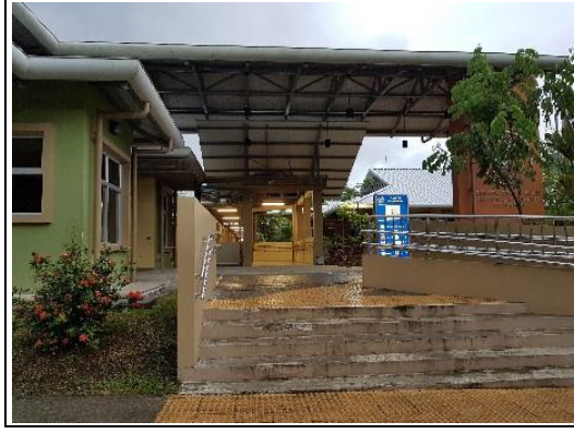
Photo 141: Entrance to new hospital in Siquirres (I-14).
