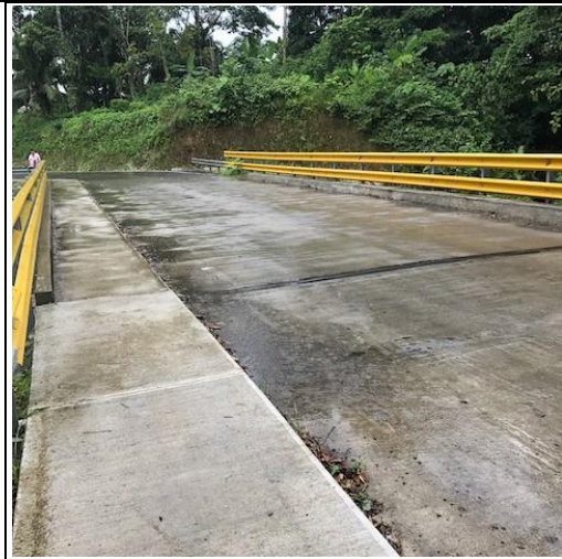
Photo 71: I-7 Bridge built over Rio Peje, between Florida and El Cruce
