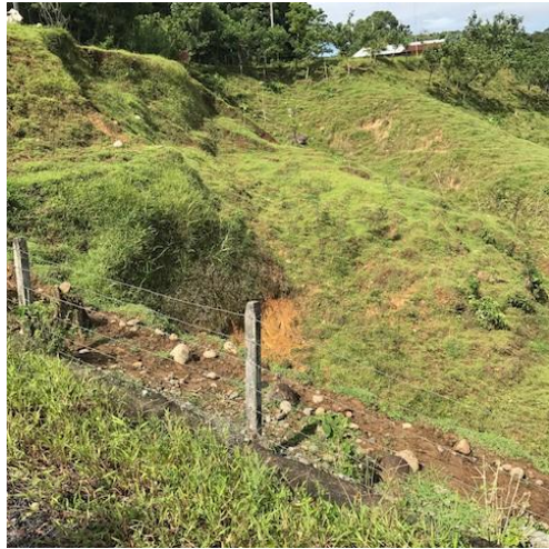
Photo 100: I-9 Farmer's land with collapsing terraces in El Coco
