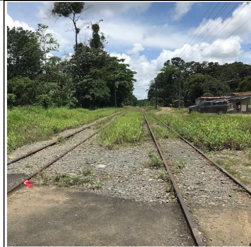
Photo 131: I-13 Remains of the historical railway in Siquirres
