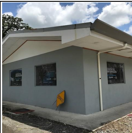
Photo 5: I-1 Communications / visitor centre under preparation at the power house site
