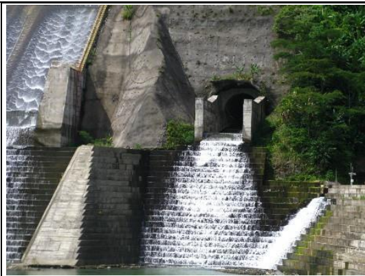
Photo 154: I-16 View of the bottom outlet
