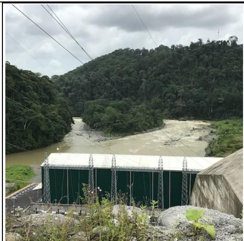
Photo 184: I-20 View downstream from immediately above the powerhouse
