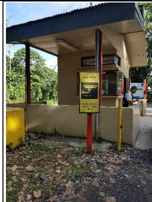
Photo 53: Video surveillance at security gates at the construction camp (I-5)
