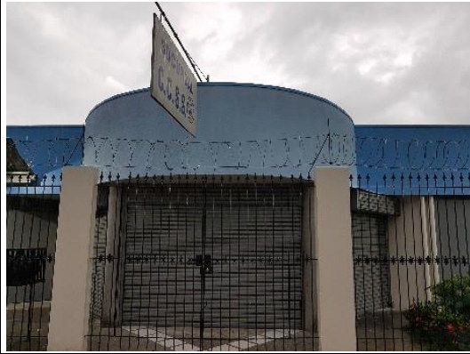
Photo 140: Public health care centre, Siquirres (I-14)
