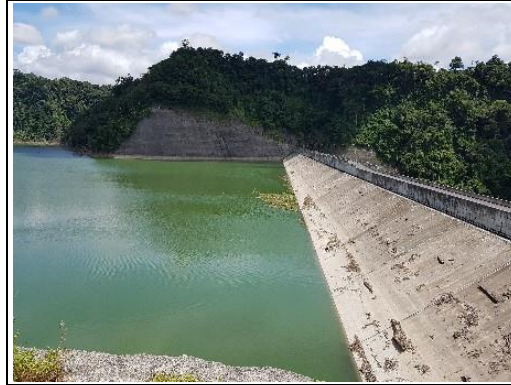
Photo 61: View of upstream concrete face of dam (I-5)
