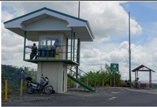
Photo 70: I-5, I-12 Security booth at the dam
