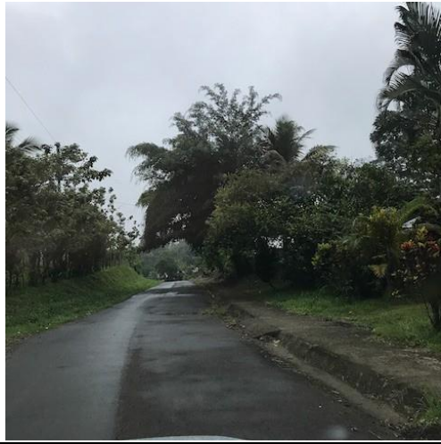
Photo 104: I-10 Road surfacing on road to Calle Nubes
