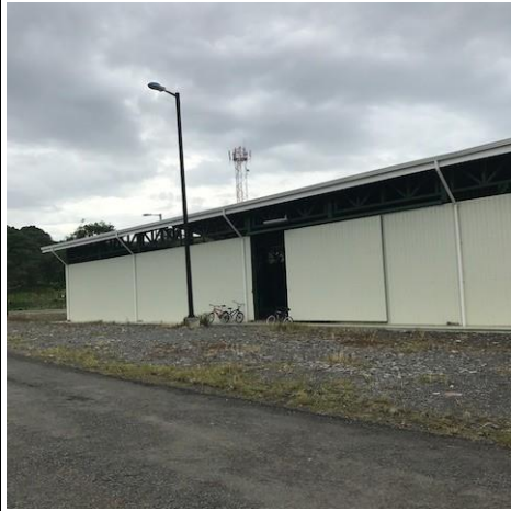
Photo 73: I-7 Sports and community hall at Florida
