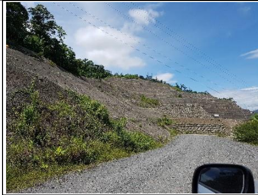
Photo 59: Slope stabilizing on right bank above spillway (I-5)
