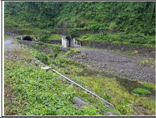
Photo 69: Outlets of diversion tunnels on left bank (I-5)
