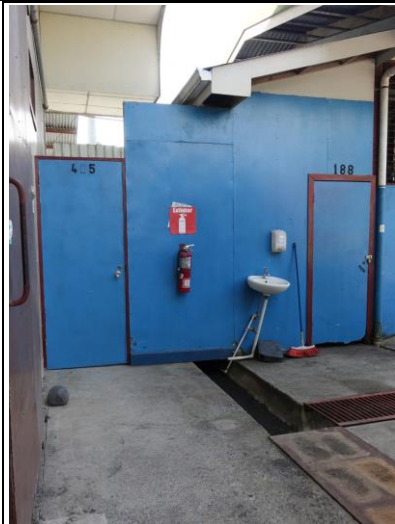
Photo 45: I-3, I-12 Drainage in camp kitchen building
