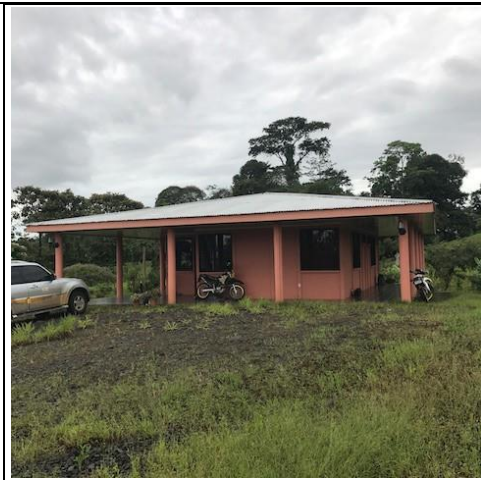
Photo 102: I-10 Replacement housing at Calle Nubes
