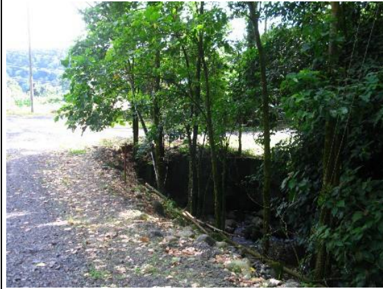
Photo 159: I-16 I-17 View of the road along Quebrada Tres Amigos
