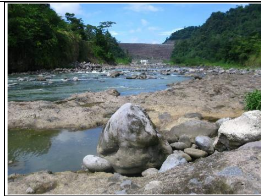
Photo 155: I-16 Boulders and cemented alluvial materials downstream
