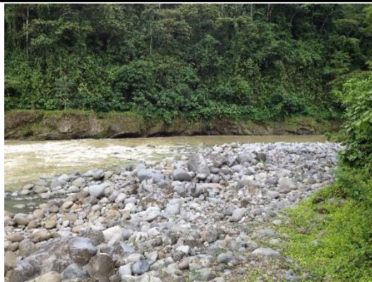
Photo 156: I-16 Banks erosion downstream before the tailrace
