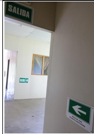
Photo 116: I-12 Safety signage in accommodation
