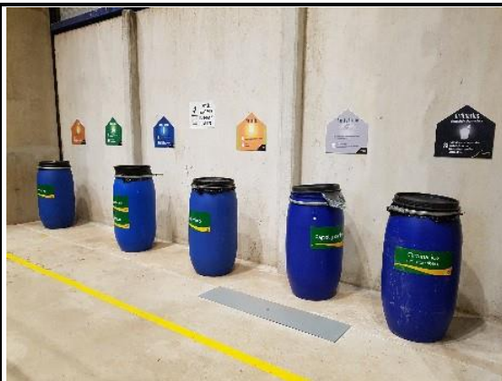
Photo 173: Waste sorting at the Reventazón power house (I-18)
