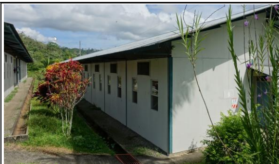
Photo 119: I-12 Workers accommodation
