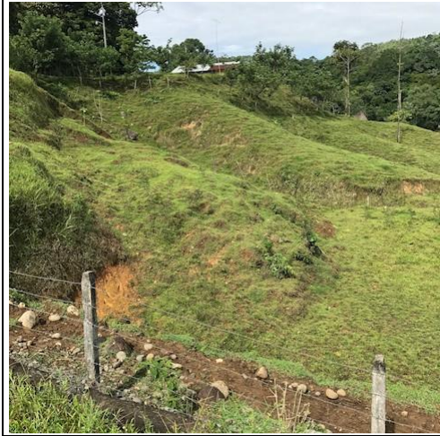
Photo 99: I-9 Farmer's land with collapsing terraces in El Coco
