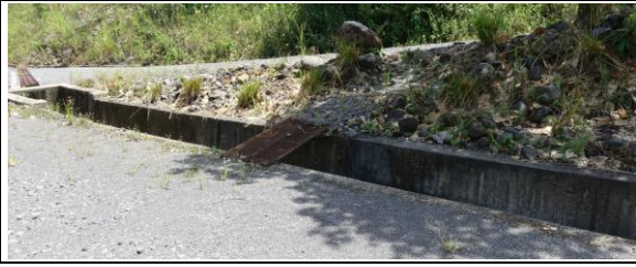
Photo 41: I-3 Site stormwater management
