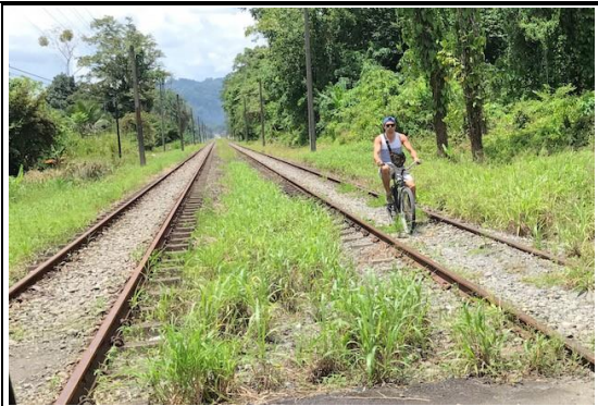
Photo 130: I-13 Remains of the historical railway in Siquirres
