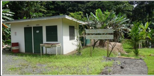
Photo 47: I-3, I-18 Wastewater treatment plant
