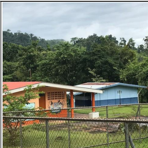
Photo 77: I-7 School classroom built at Pascua (the blue building)
