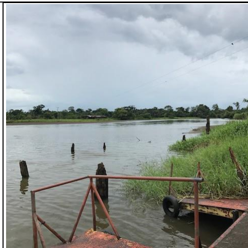
Photo 195: I-20 View of Reventazón River at Cano Blanco / Parismina
