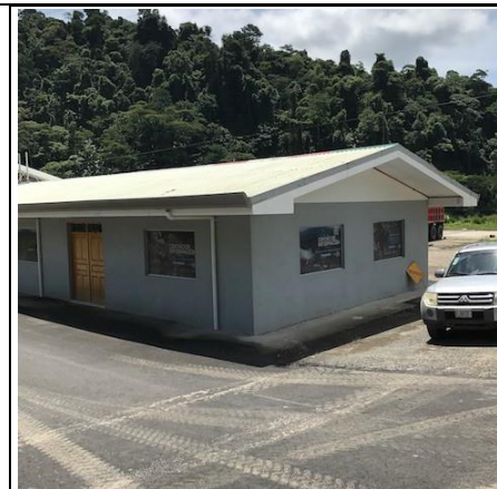
Photo 6: I-1 Communications / visitor centre under preparation at the power house site
