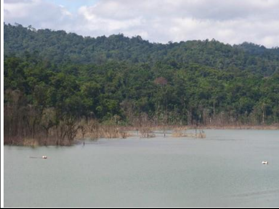
Photo 174: I-19 View of the reservoir shore from the dam and safety buoys
