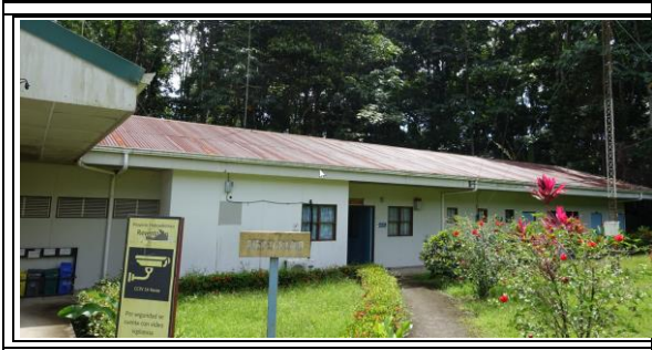
Photo 121: I-12, I-14 Health centre on site
