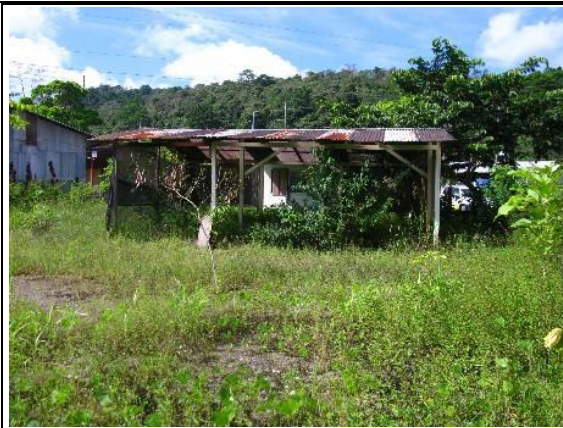
Photo 150: I-15 Disused nursery on site
