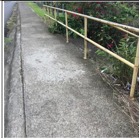
Photo 91: I-9 Sidewalk built in Florida to minimize public exposure to project traffic, with railing to minimize falling hazard
