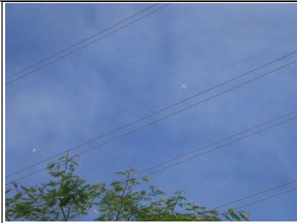
Photo 149: I-15 Measures to prevent birds collision on transmission lines
