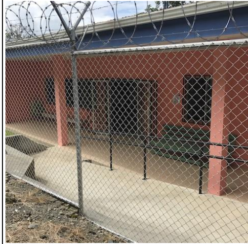
Photo 80: I-7 EBAIS building at Santa Marta
